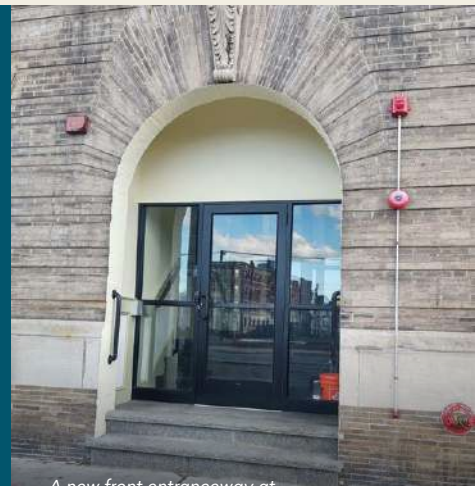
A new front entranceway at 1202 Commonwealth Ave in Allston
