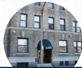
ALLSTON Commonwealth Ave.
